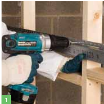
2 Resilient Bar fixed to one side
